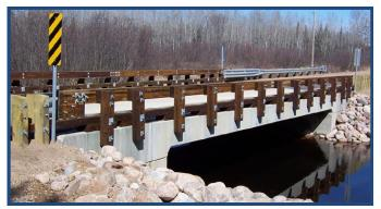
All timber materials are pressured treated and all hardware is hot-dipped galvanized. Appropriate material certifications are available.
